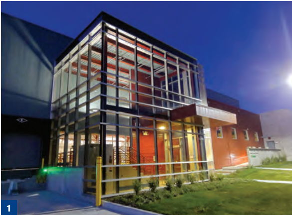
1. Completed NOvA experiment building in Minnesota. 2. The roof uses a six-inch layer of barite, which is 60 percent heavier than a six-inch layer of common granite, to shield the detector inside from cosmic rays. NOvA is a two-detector experiment with the smaller of the two, a 200-ton “near detector,” at Fermilab, and a 15,000-ton “far detector” 503 miles away in Ash River, Minn.
