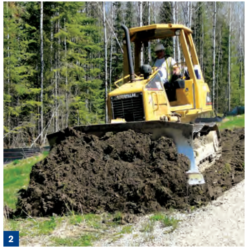
1. The experiment involves about 180 scientists and engineers from 28 institutions. 2. Rock removed to dig a 40-foot-hole to house the detector and building was repurposed for the site's berm and road. 3. Interior of the detector hall. The detector will be installed in 2012. 4. The building housing the NOvA far detector, which weighs as much as 150 fully loaded school buses.
