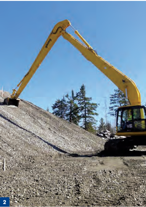
1. The experiment involves about 180 scientists and engineers from 28 institutions. 2. Rock removed to dig a 40-foot-hole to house the detector and building was repurposed for the site's berm and road. 3. Interior of the detector hall. The detector will be installed in 2012. 4. The building housing the NOvA far detector, which weighs as much as 150 fully loaded school buses.
