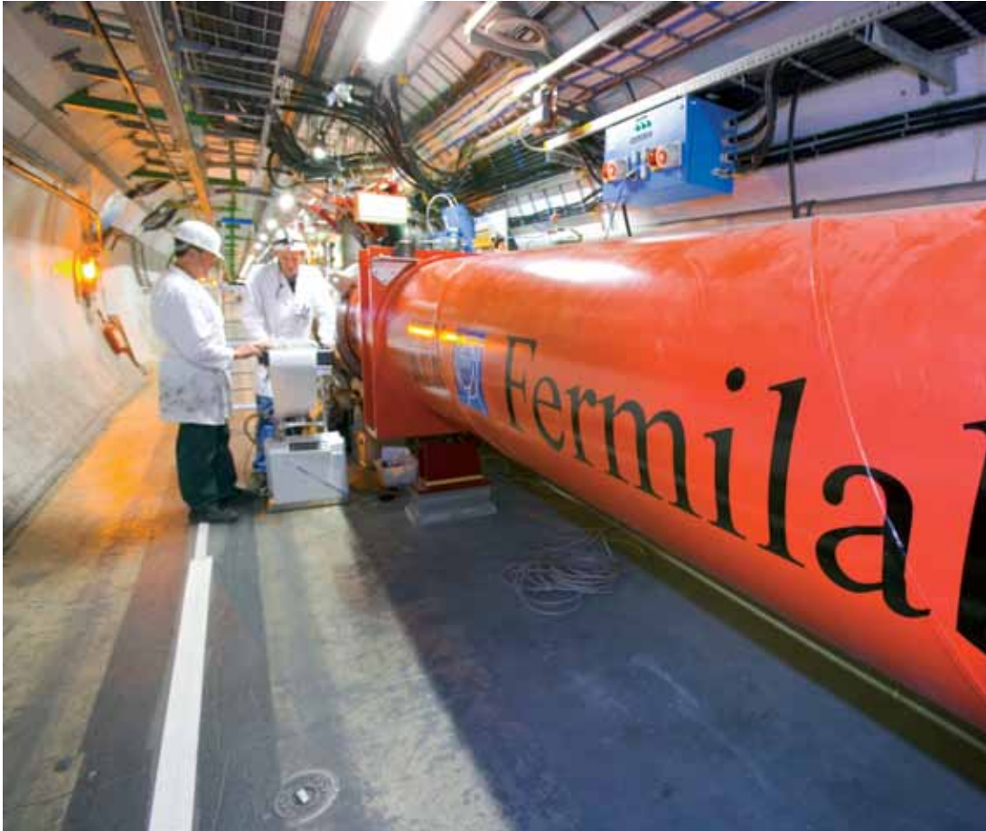
Scientists and engineers from Fermilab and from Japan's KEK laboratory designed, built and shipped advanced high-tech quadrupole magnets to Switzerland for the Large Hadron Collider accelerator at CERN. Can future accelerator builders go beyond this level of worldwide contribution to become truly international efforts from the start?
