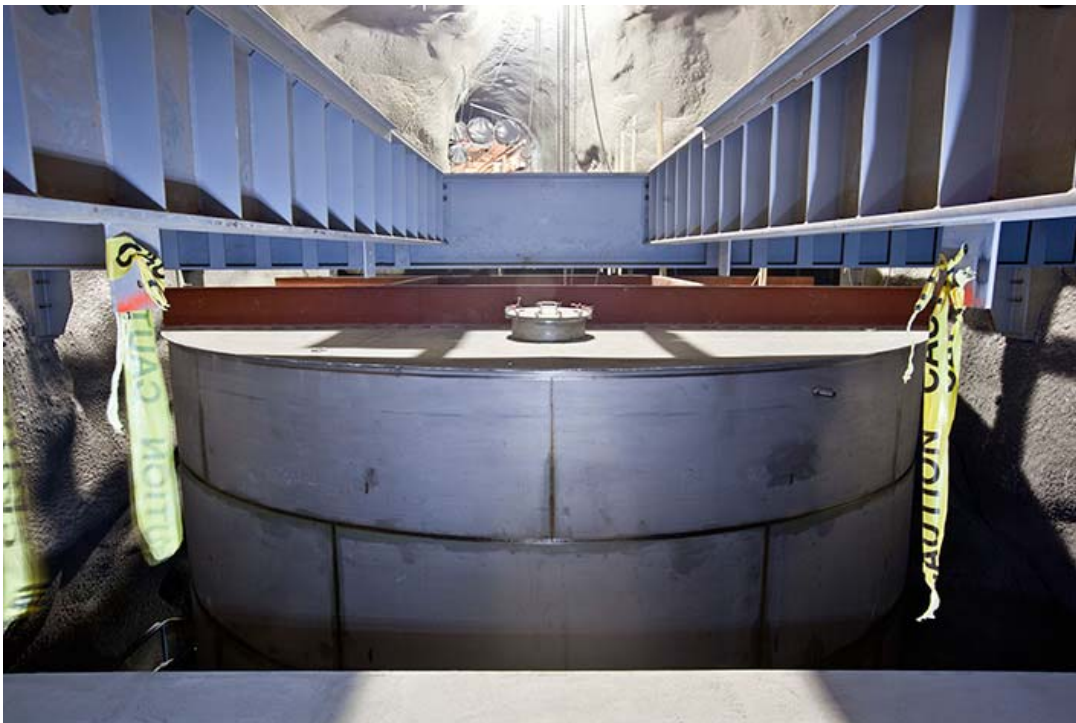
The stainless steel tank, completed in January 2011, will hold 71,600 gallons of purified, deionized water to protect the LUX detector from naturally occurring radioactive decays. Technicians will lower the detector into the water this summer. Photo: Matt Kapust
