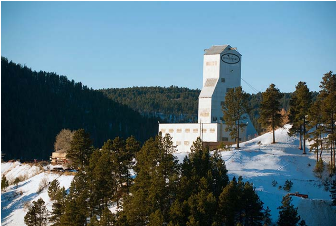
The Homestake mine in South Dakota, known for its iconic headframes and a depth of more than 8000 feet, closed in 2003. The state of South Dakota began reopening the mine for science in 2007. Photo: Reidar Hahn
